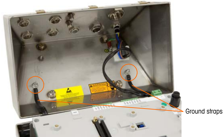
Figure 2-9: Loosening the Ground Straps
