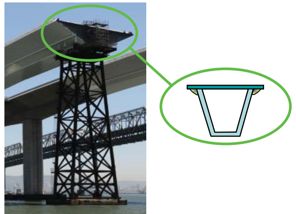
The new San Francisco Bay Bridge uses closed orthotropic ribs similar to the ribs used in our weighing bridges.
