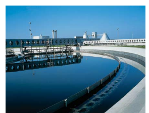
Wastewater process: biological water treatment.
