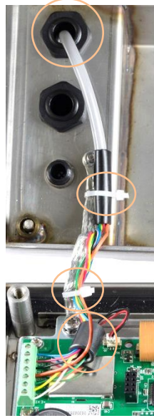
Figure 2-28: Analog Load Cell Pin Grounding and Ferrite Installation, IND236
