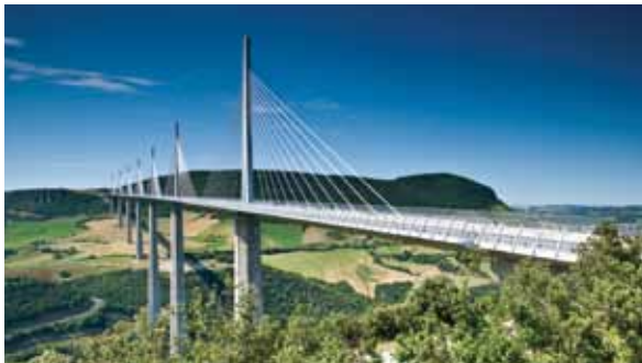
The Millau Viaduct in France relies on orthotropic ribs for its structural support.
