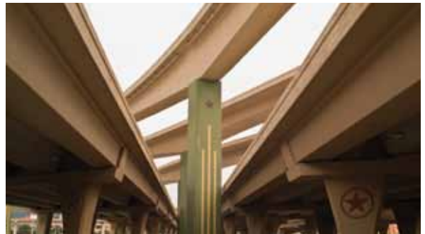
Orthotropic ribs are used in the High Five interchange in Dallas, Texas.
